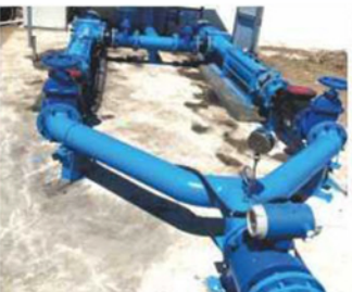
Screw pump is used to transport aquaculture wastewater
