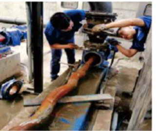
Sewage plant screw pump accessories replacement
