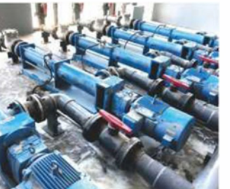
Sludge circulating pump of sedimentation tank
