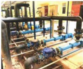
Screw pump is used for sludge in sedimentation tank
